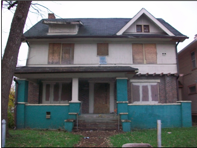
Before photo of 3028 Park Avenue
