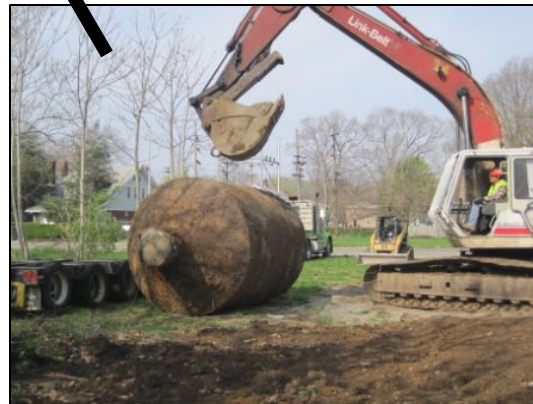
2 USTs Removed (100 & 4,000 gal) from Former Dry Cleaners Site
