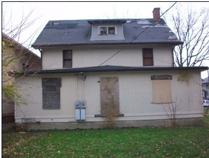
Before photo of 3028 Park Avenue
