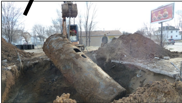
7 USTs Removed (from 750 to 3,000 gal) from Former Gas Station Site
